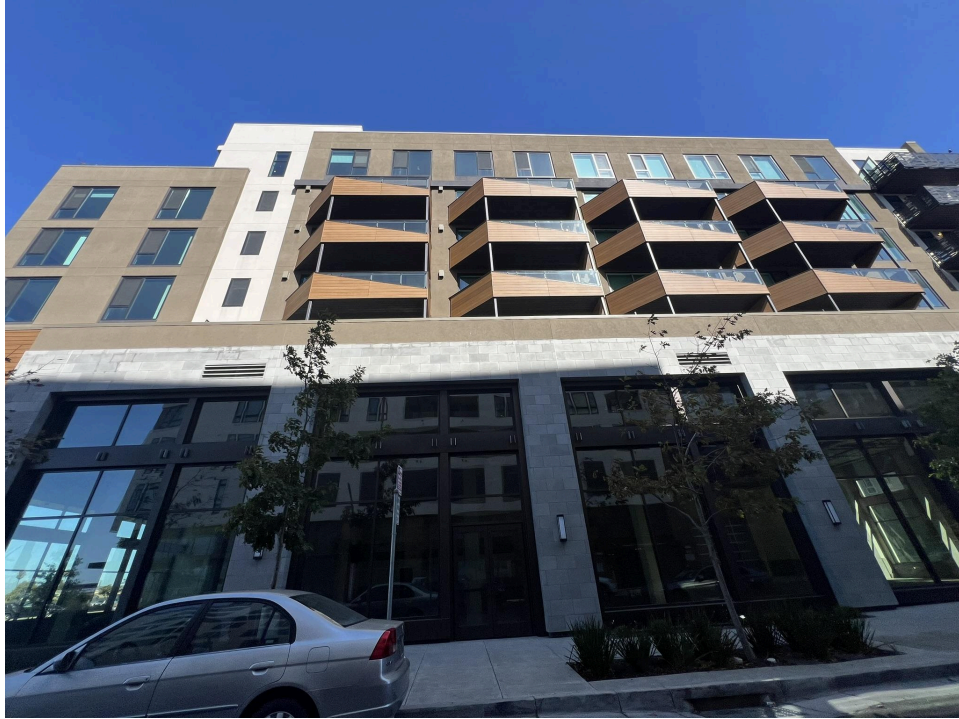
Parcel G (Caspian) Completed
