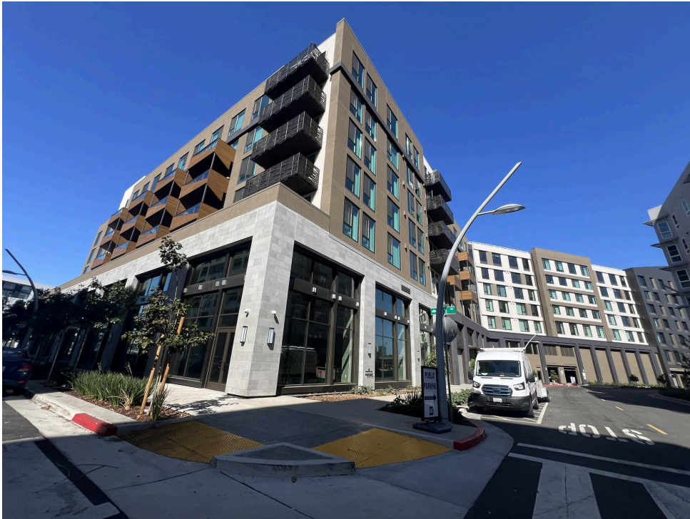
Parcel G (Caspian) Completed
