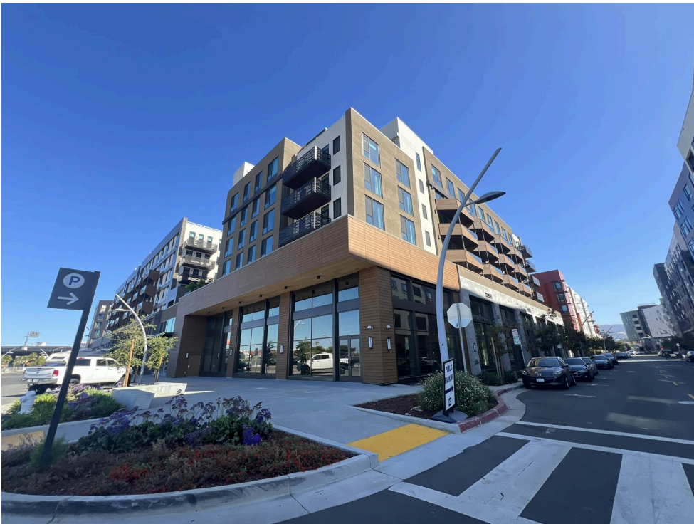
Parcel G (Caspian) Completed
