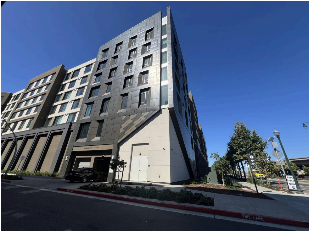
Parcel G (Caspian) Completed
