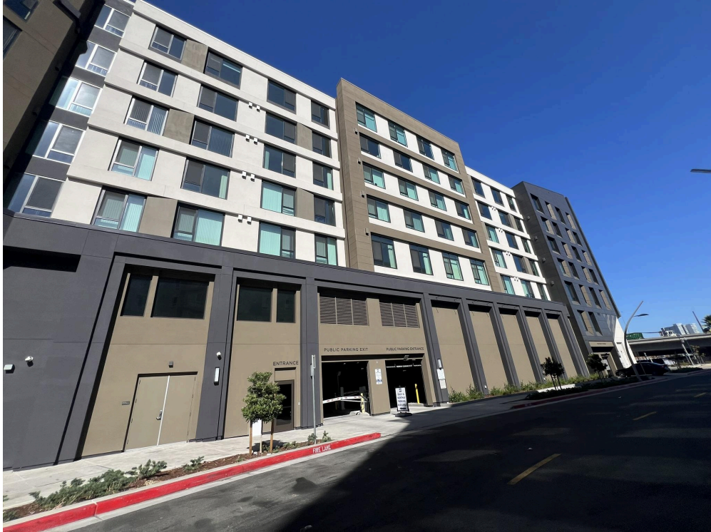
Parcel G (Caspian) Completed
