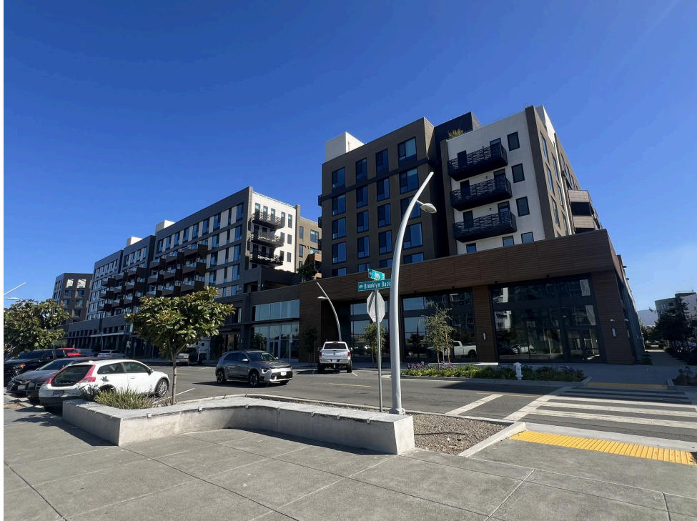
Parcel G (Caspian) Completed
